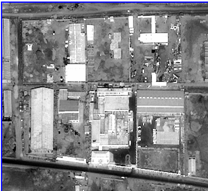
FIGURE 8: Shifa pharmaceutical plant, Sudan.
